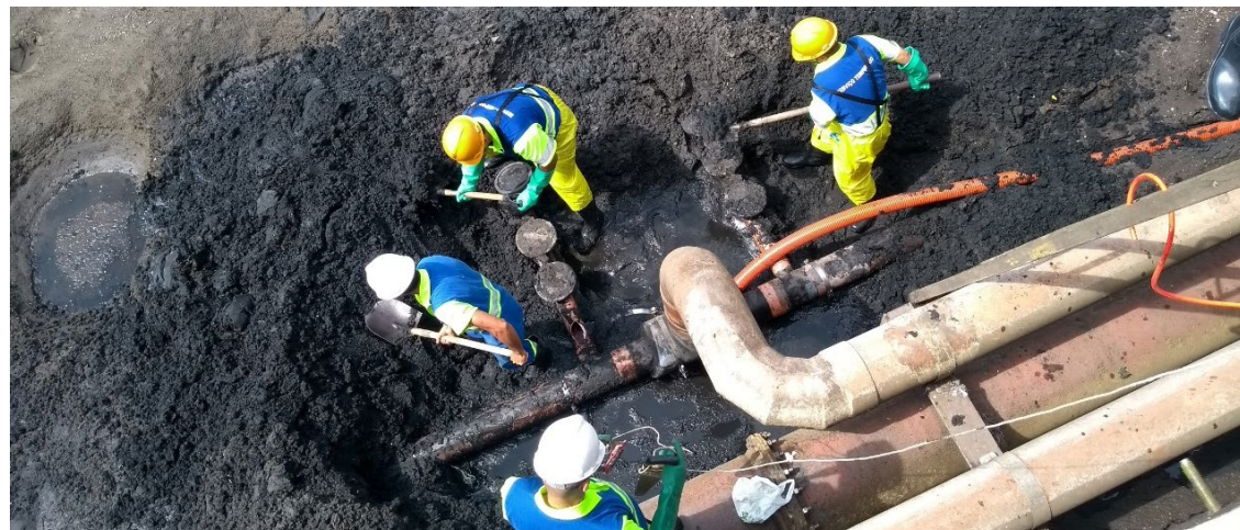
Team promotes improvements in the Porto Novo sewage treatment plant, in Caraguatatuba (North Coast)
