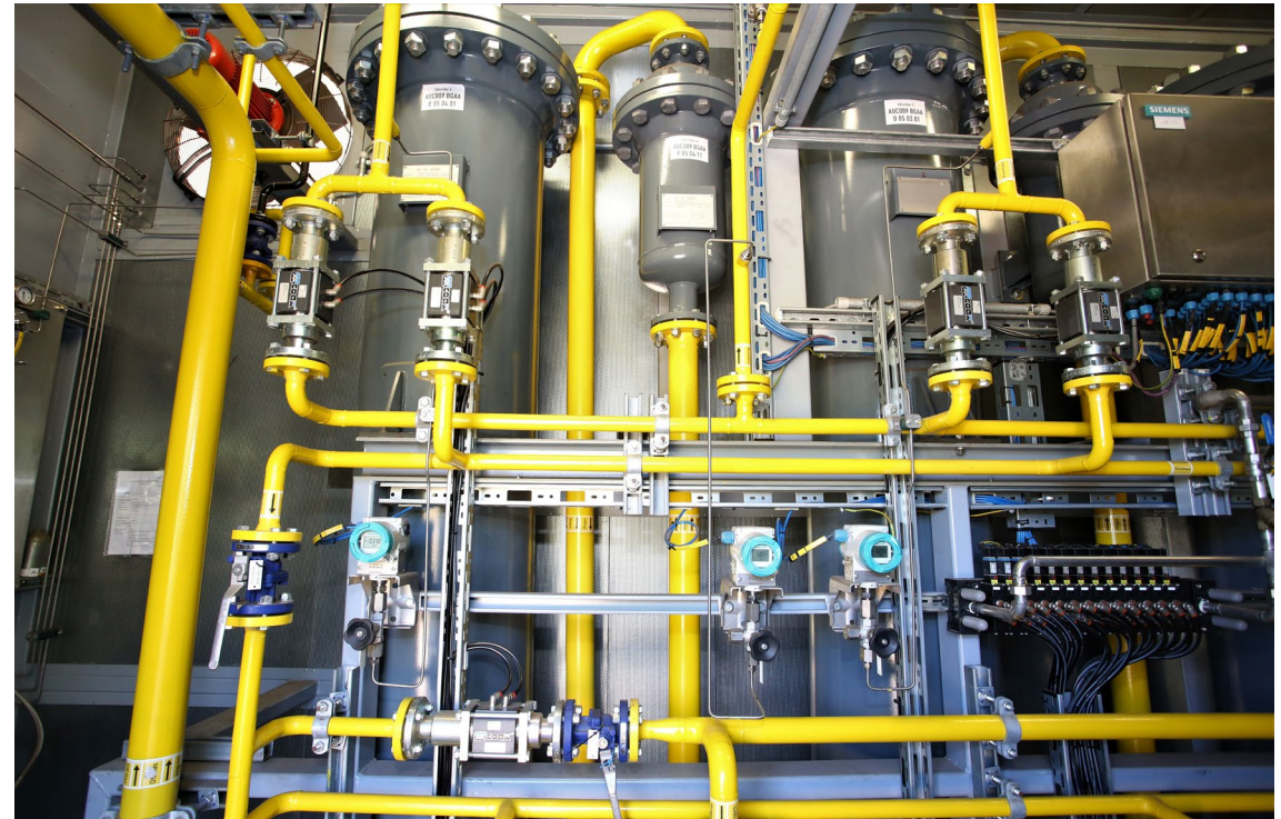
Biogas generated at the Franca STP is transformed into biomethane fuel to supply the local vehicle fleet
